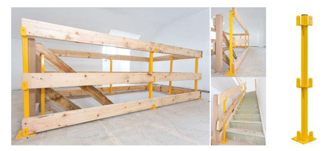
Steel posts provide secure support for temporary edge protection to staircases and landings during construction
